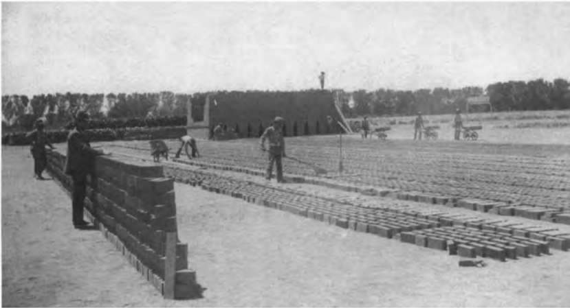
Adobe remained a popular and economical building material in Phoenix well into the twentieth century. This scene of an adobe plant shows the process of forming and drying bricks. A test wall stands at the left of the image. Boudoir cabinet card, F. A. Hartwell photographer, ca. 1895.
